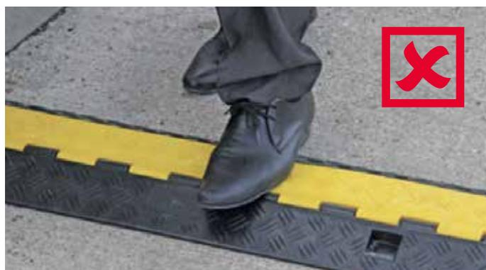
**Figure 4. Cable protectors sit on top of the cable. This is still a health and safety hazard and is not permitted.**
