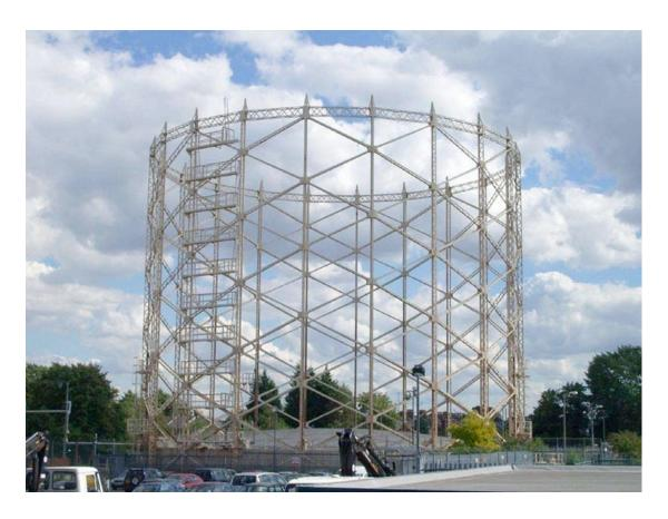
What makes this structure so important is its highly innovative design that uses helical (or spiral-like) girders joined to vertical members to form triangular cells with each side being equally stressed. This provides for a very strong yet relatively light weight structure with the vertical elements also acting as guide rails for the gas tanks
